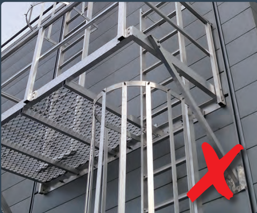
Certified by an engineer, Defender landings are installed with the correct structural fixings and never Tek screwed into flashing.
