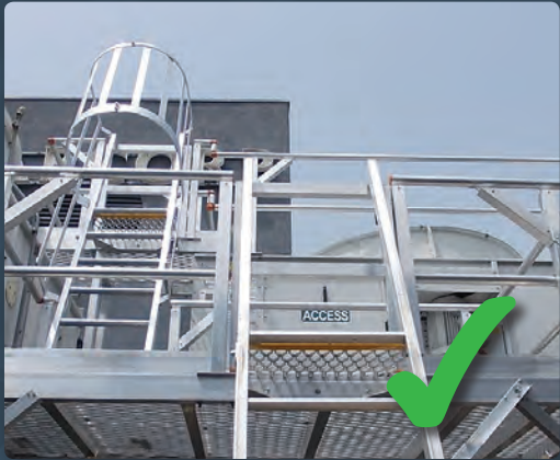
Defender landings & platforms are the correct size with proper clearances and mounted structurally rather than merely on the ladder stile.
