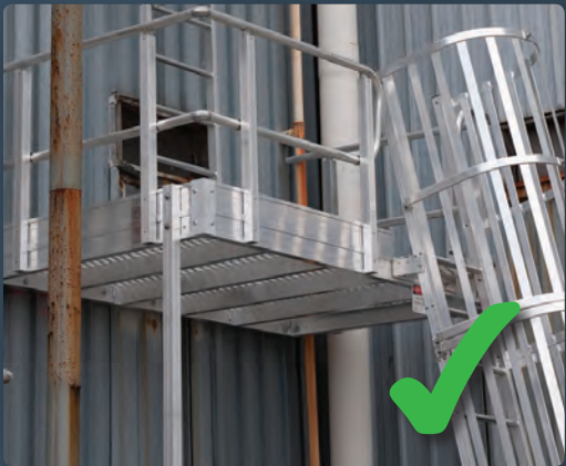
Certified by an engineer, Defender landings are installed with the correct structural fixings and never Tek screwed into flashing.
