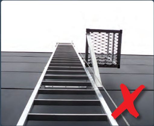
Defender landings & platforms are the correct size with proper clearances and mounted structurally rather than merely on the ladder stile.
