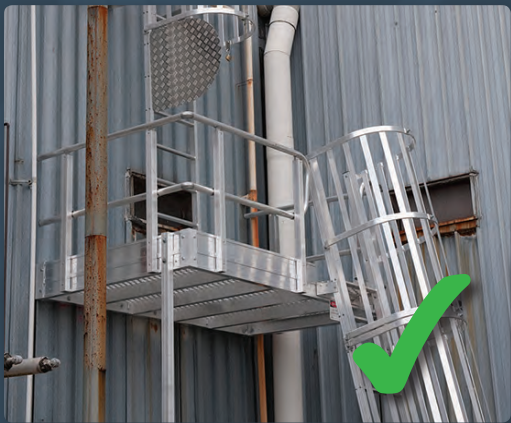
Defender is load-rated to 2.5kPa (for two-person use) and certified by CodeMark™ to the installation standard with full compliance to the National Construction Code.
